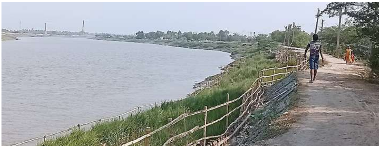
Fencing at Ghoshpur Site
