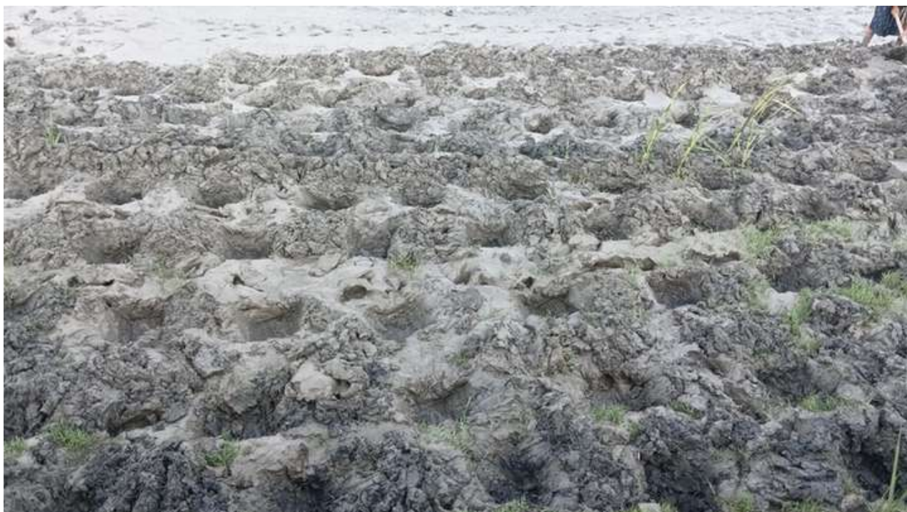
Digging of pits
