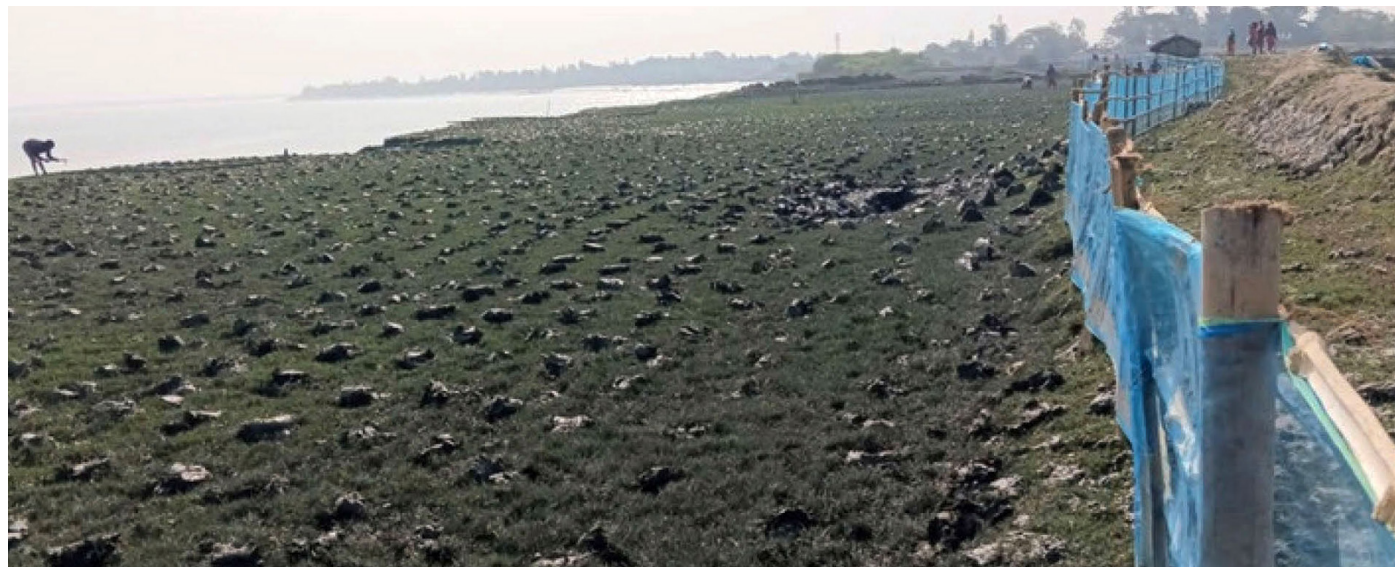
Digging of pits
